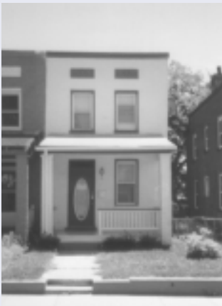
1835 L Street NE, after renovation
